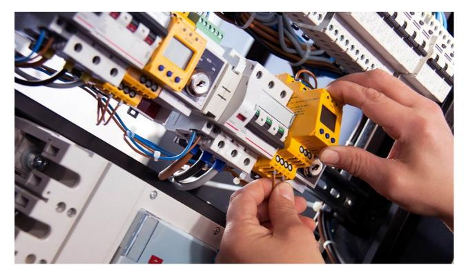
As you may know, MCBs are tiny devices that act as controlling agents during an unusual supply of power. This mechanism cuts off an electrical system as soon as it detects an overload or a power surge. Generally, it finds use as a replacement for a fuse. Depending upon the nature of the electrical applications, you can incorporate different types of MCB in your residences and in industries. Read this new blog in Linquip to find out more about them.
