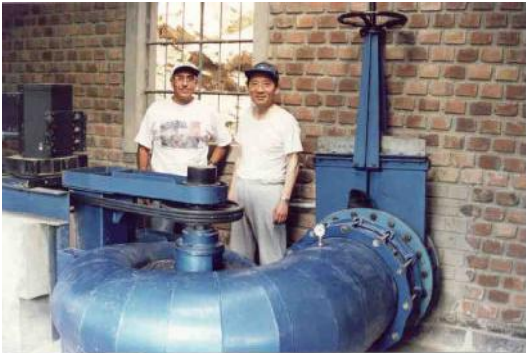
Figure 19. ITDG spiral Kaplan turbine
