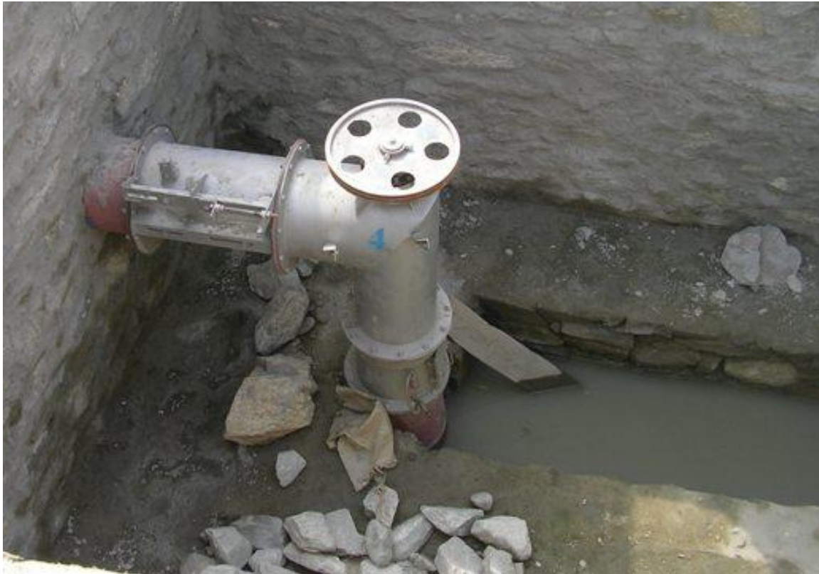
Figure 5. Kaplan turbine being installed, note water level in tail race
