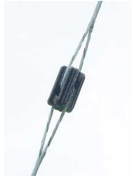
Stay Insulator (Reference: electricaleasy.com )
