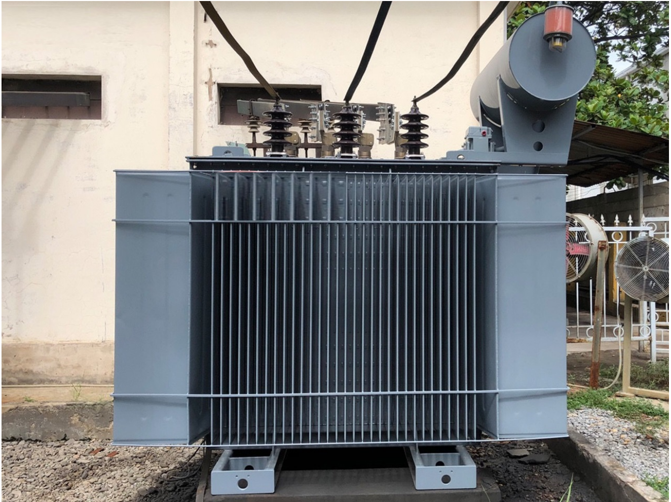
Step Up Transformer in Power Distribution (Reference: vietnamtransformer.com )
