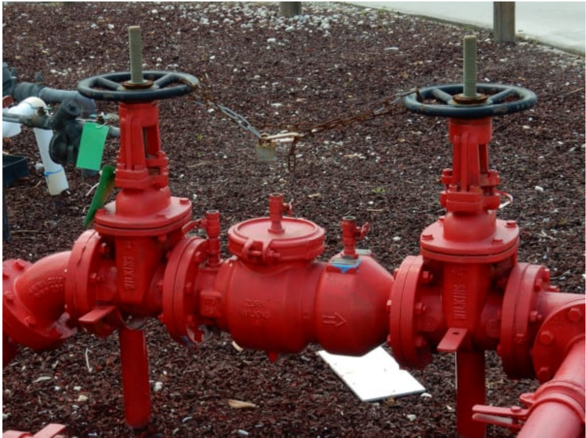
A backflow preventer (Reference: qrfs.com )
