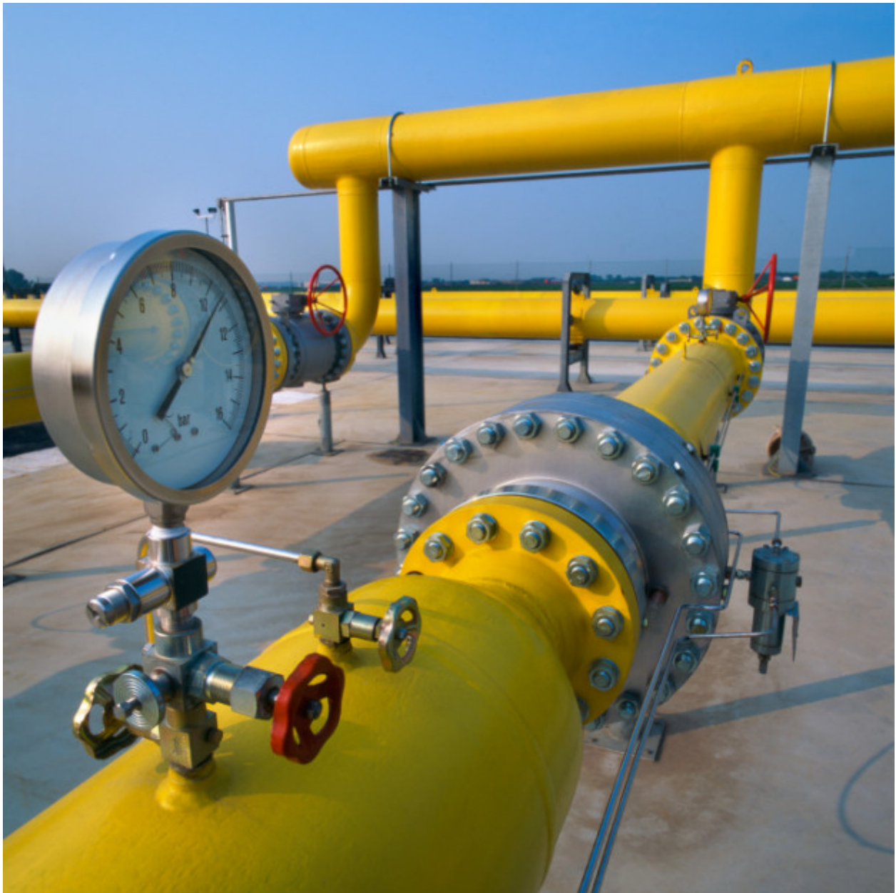
Hydro testing (Reference: binfraih.com )
