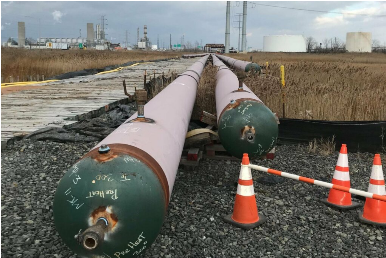
Pipeline pre-commissioning (Reference: americanpipelinesolutions.com )
