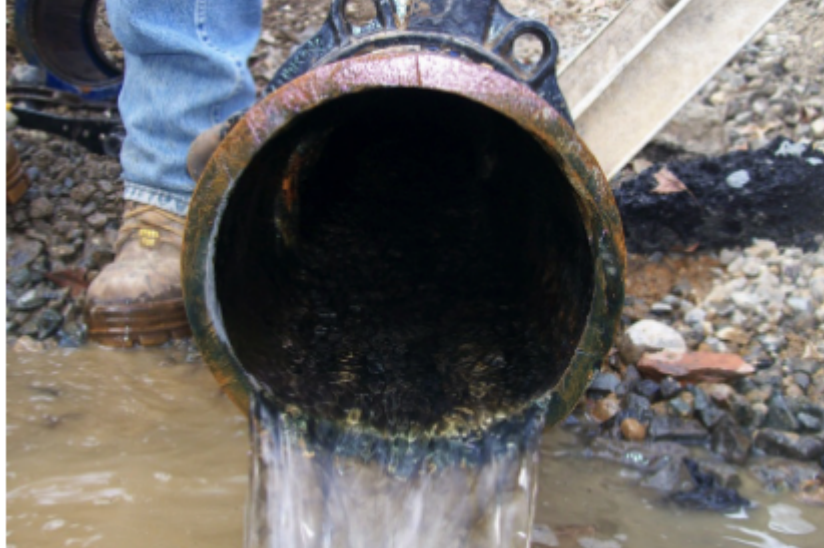
Dewatering (Reference: americanpipelinesolutions.com )
