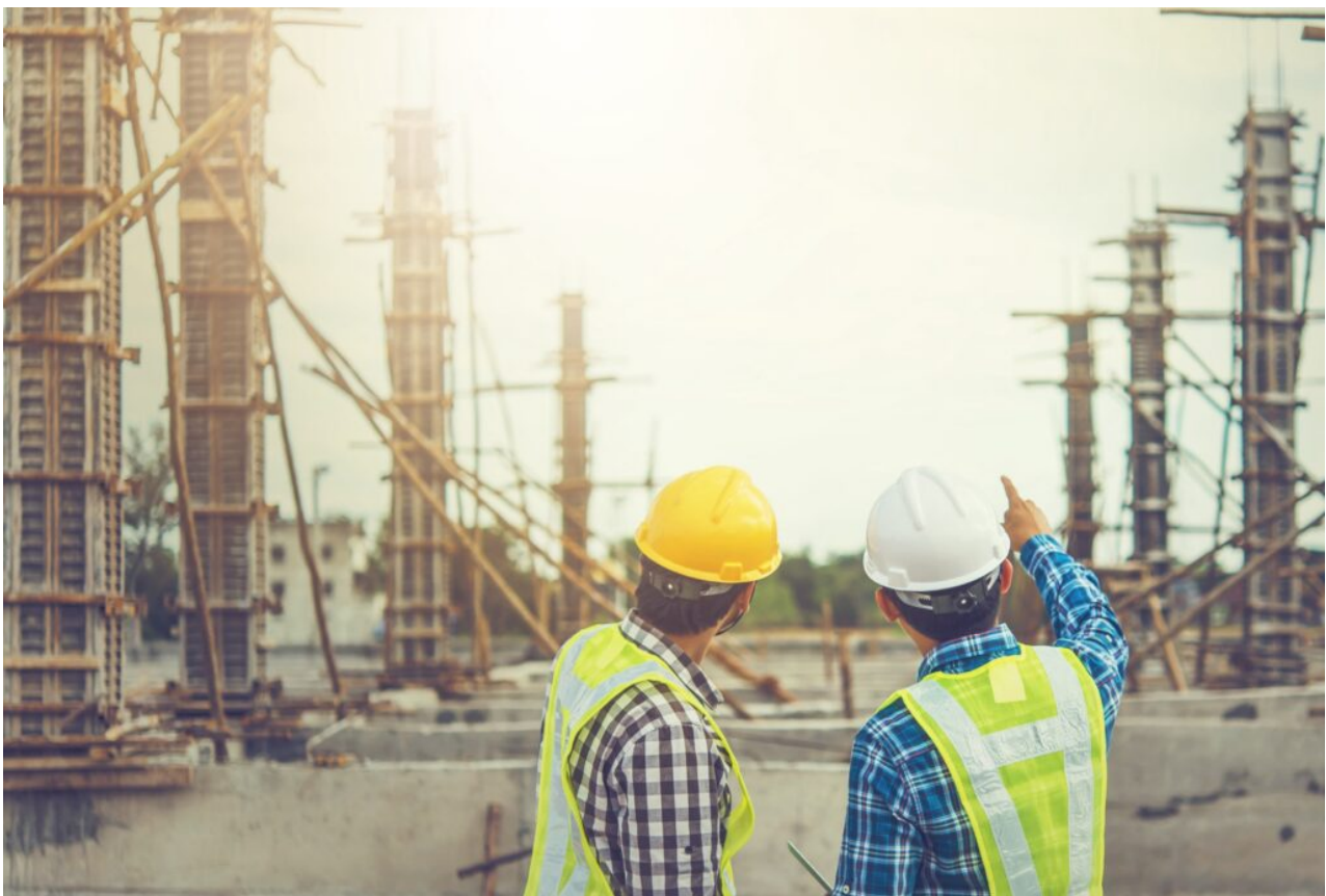
Civil engineering (Reference: ncl.ac.uk )
