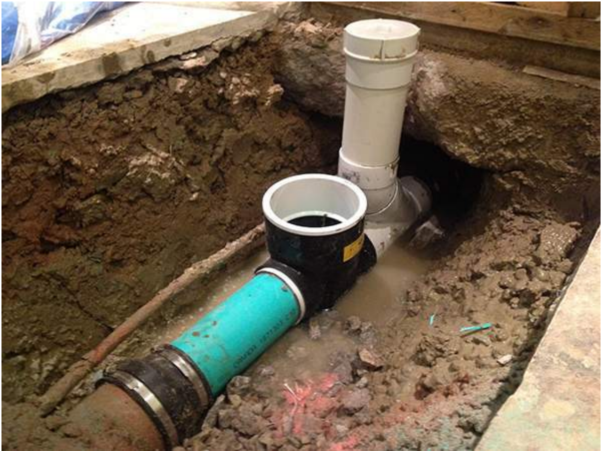
Installation of a backwater valve (Reference: mydecorative.com )
