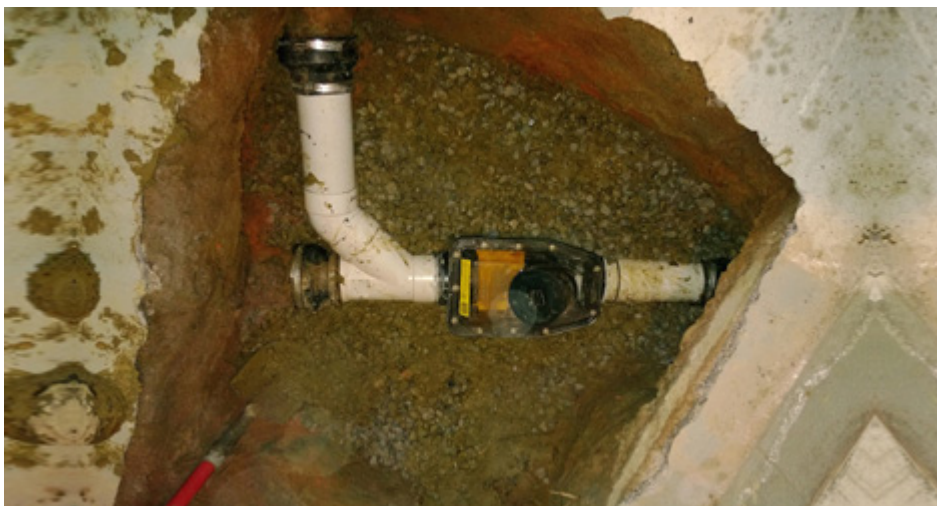
Backwater valve maintenance (Reference: themapleroots.com )
