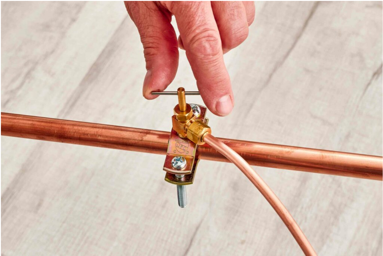
Installation of a saddle valve (Reference: thespruce.com )
