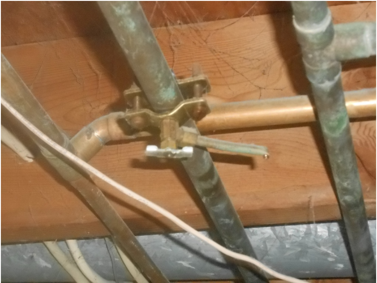
Fixing the leak at a saddle valve (Reference: diy.stackexchange.com )
