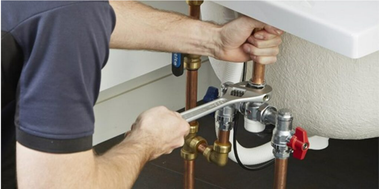
Thermostatic mixing valve maintenance (Reference: sms-environmental.co.uk )
