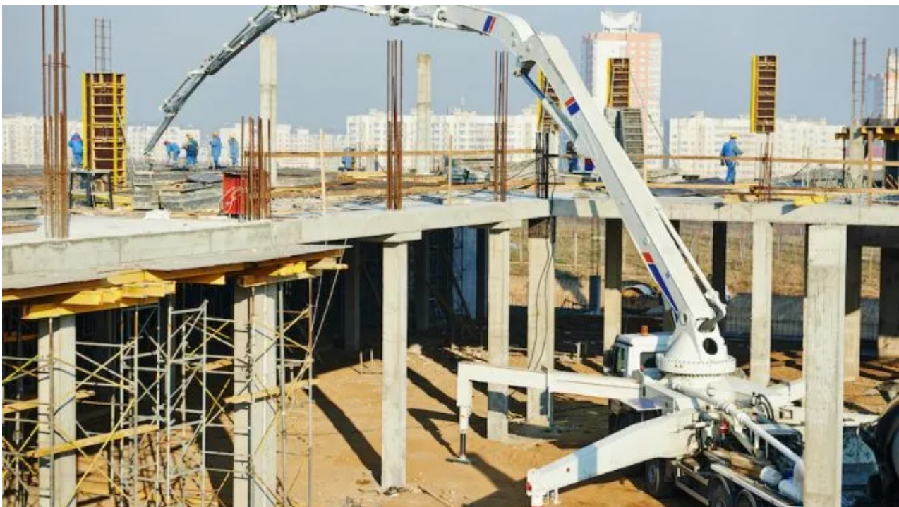
Application of concrete pump (Reference: civiconcepts.com )
