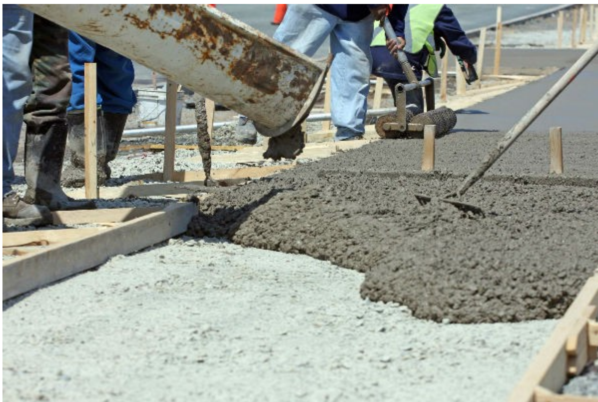
Ready mix concrete (Reference: constrofacilitator.com )
