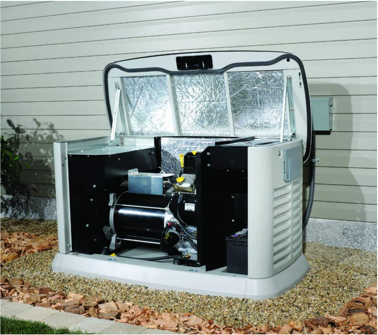
Standby generator installation (reference: blog.norwall.com )
