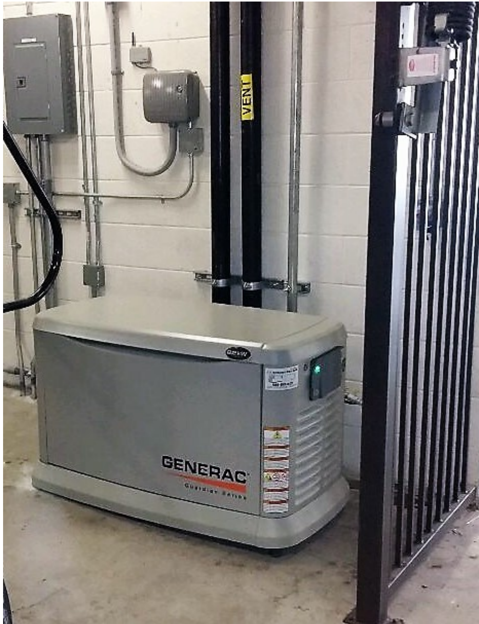
Installation of a 22kW Generac generator (Reference: ltgenerators.com )
