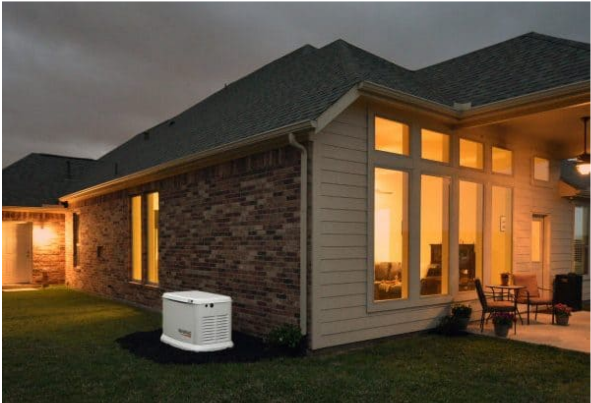
Standby generator (Reference: blog.norwall.com )
